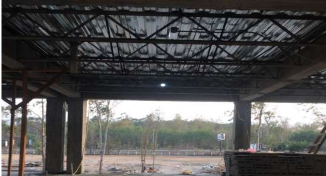
Colocado de Joist
