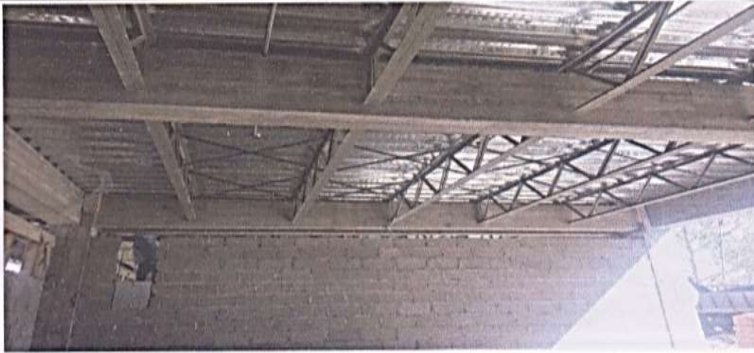
Colocado de Joist
