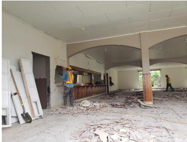
**DESMONTAJE DE CIELO FALSO PANELIT EN MAL ESTADO EN EL AREA DE COMEDOR**
