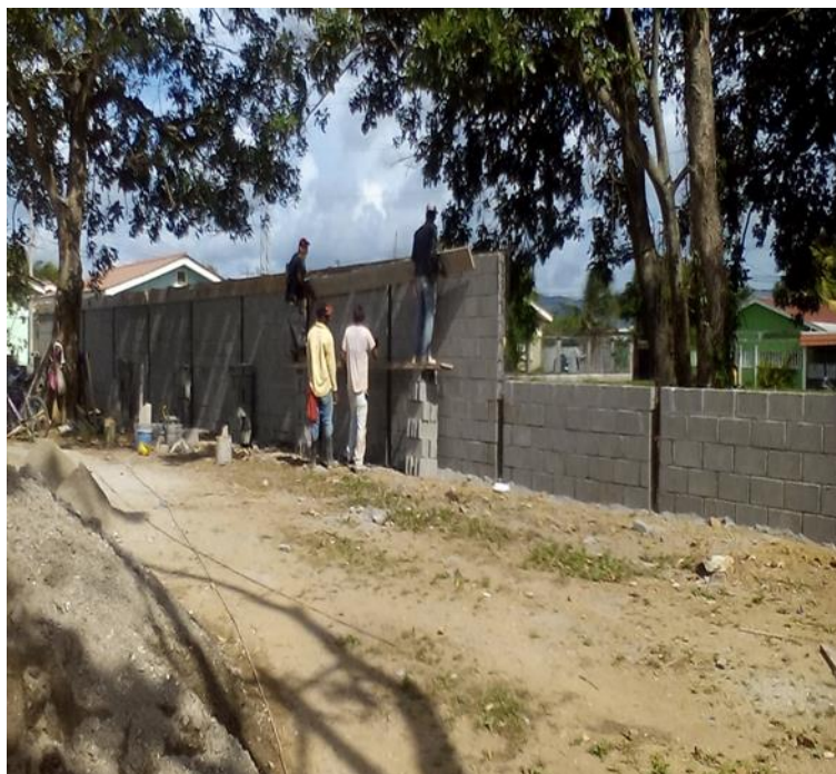
8 Supervision cerco perimetral I.H.S.S.
