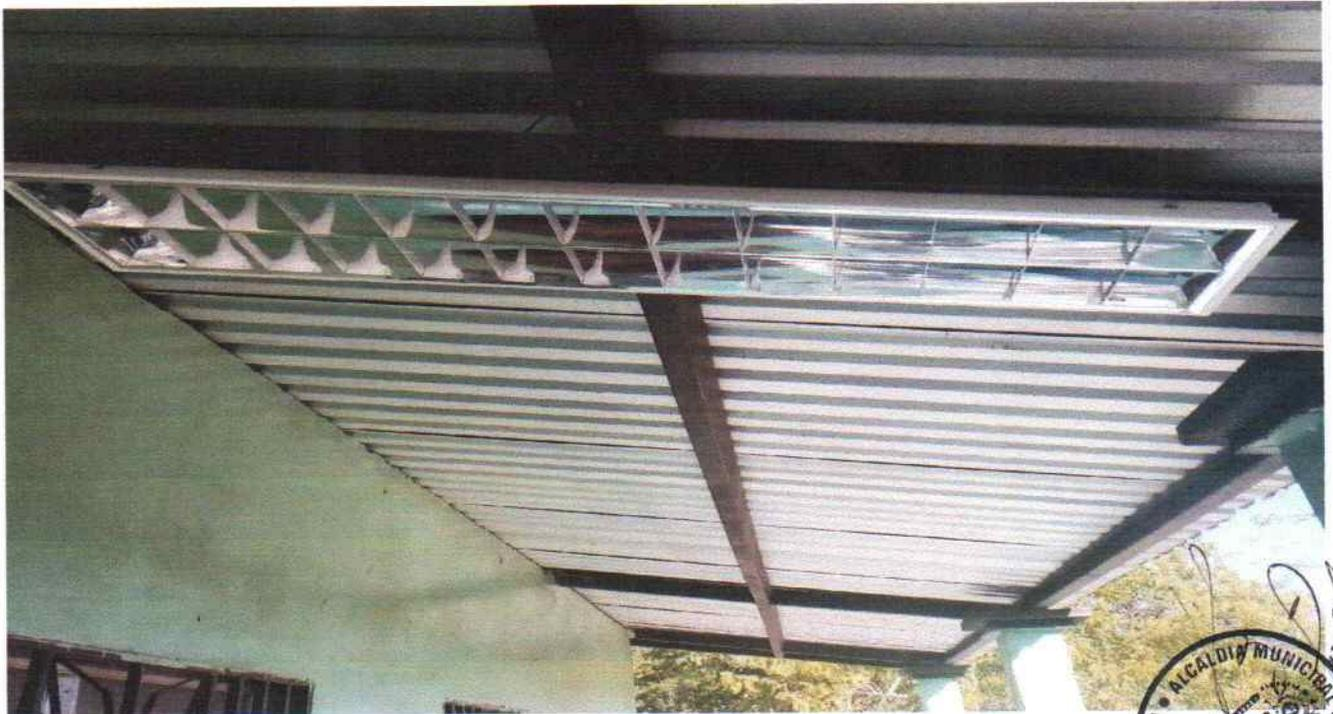
Figura No.2, Lámparas led Instaladas
