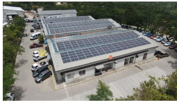
Perspectiva General de naves, COPECO-Central
